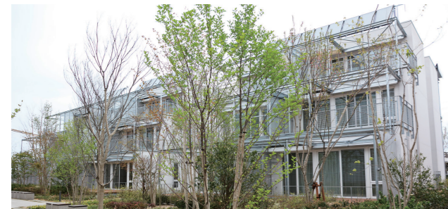
View of the Passive Town Block No. 1. The panels visible near the top of the outer walls collect solar heat for water heating.
