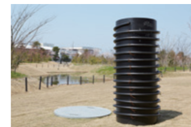
A heat exchange system at the Maruyane Exhibition Hall
