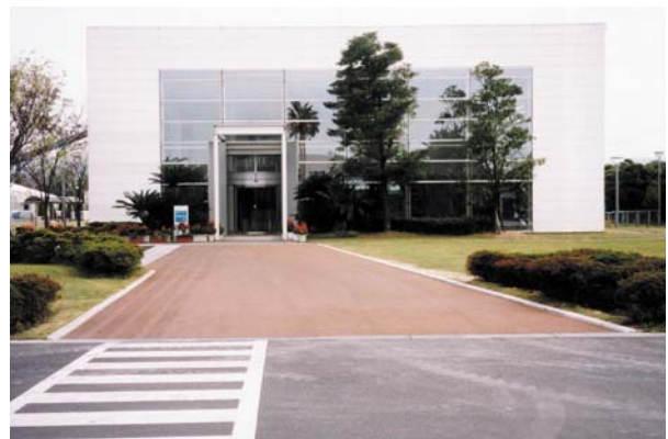
Kyushu factory: Glass was converted to roadway subgrade material and used on the YKK company grounds.
