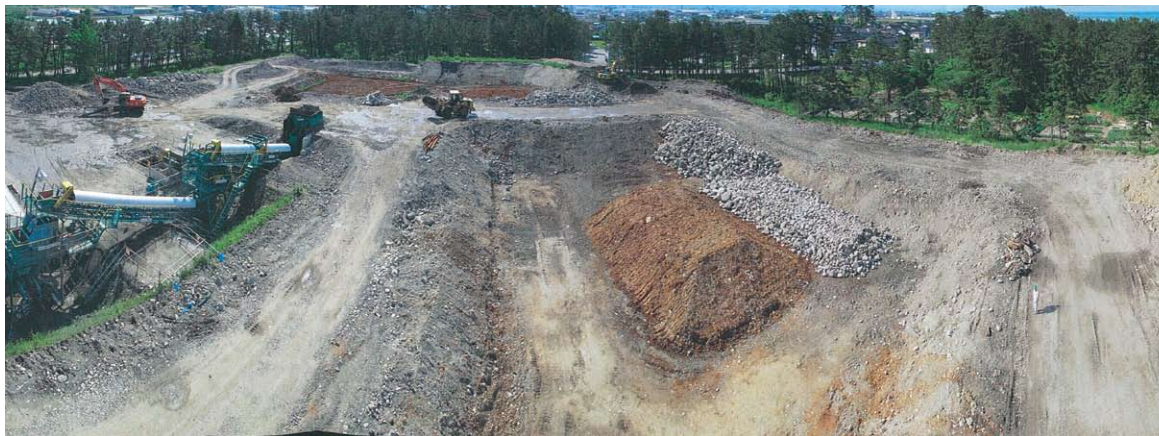
Clearing of landfill and reclamation of land
