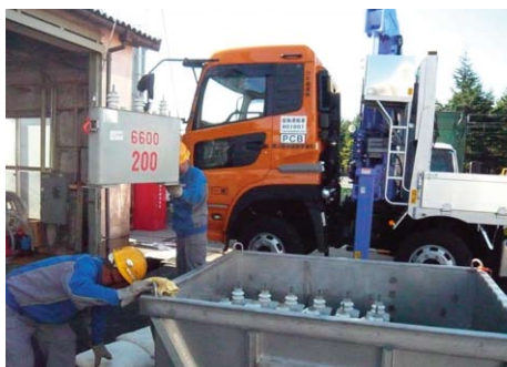
Transport of equipment containing high concentrations of PCBs to disposal facility
