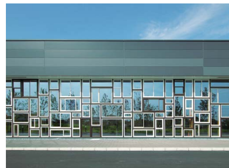
YKK AP Saitama MADO (window) Plant
