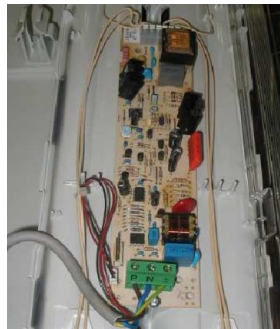
YKK ITALIA S.P.A. We installed energy-saving lights throughout the plant (3,570 in all) that automatically adjust brightness levels according to the amount of natural light coming in.
